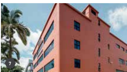
7 31 Changi South Avenue 2
