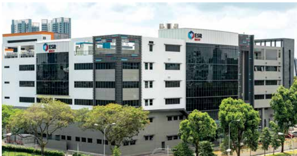
30 Marsiling Industrial Estate Road 8 ◀
