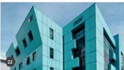
22 45 Changi South Avenue 2
