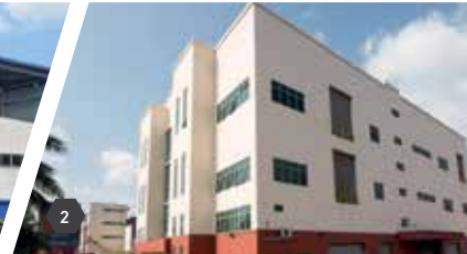
2 79 Tuas South Street 5
