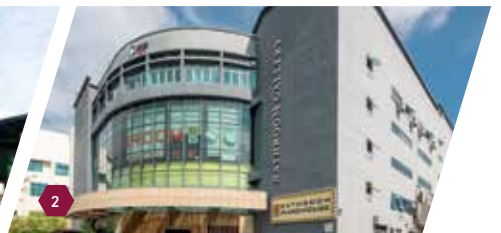
2 25 Changi South Avenue 2
