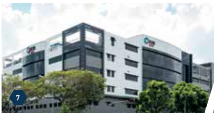
7 30 Marsiling Industrial Estate Road 8
