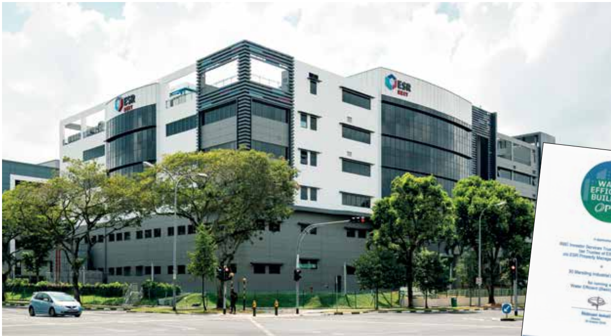
30 Marsiling Industrial Estate Road 8
