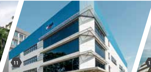
11 60 Tuas South Street 1
