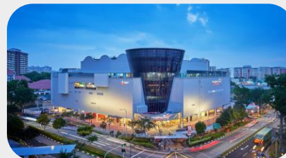
Completion of Hougang Mall AEI at ROI ~8%
