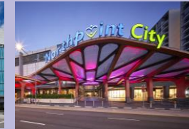
Northpoint City North Wing
