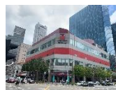
Cross Street Exchange
