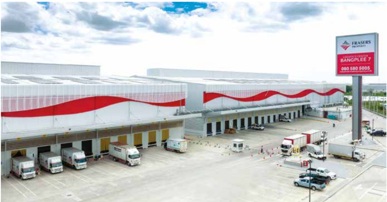
Fraser's Property Logistic Center (Bangplee 7), Samut Prakan, Thailand
