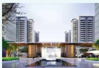
Completed and settled residential development Palace of Yunjian, Shanghai, China, 4Q FY24
