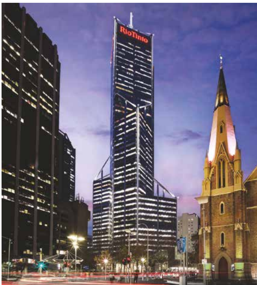
Central Park, Perth, Western Australia
