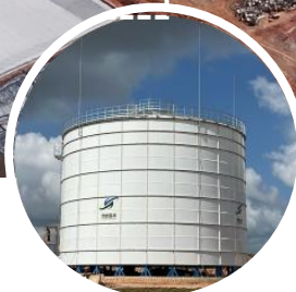
Bio-digester & Manure Treatment & Biogas Generator
