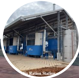
Feed Storage and TMR System Ready
