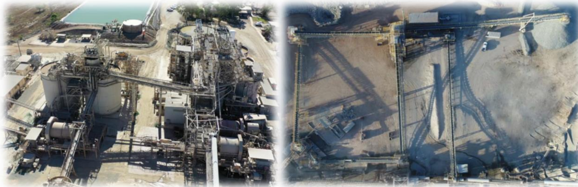
Processing plant with the grinding mill and beneficiation circuit
