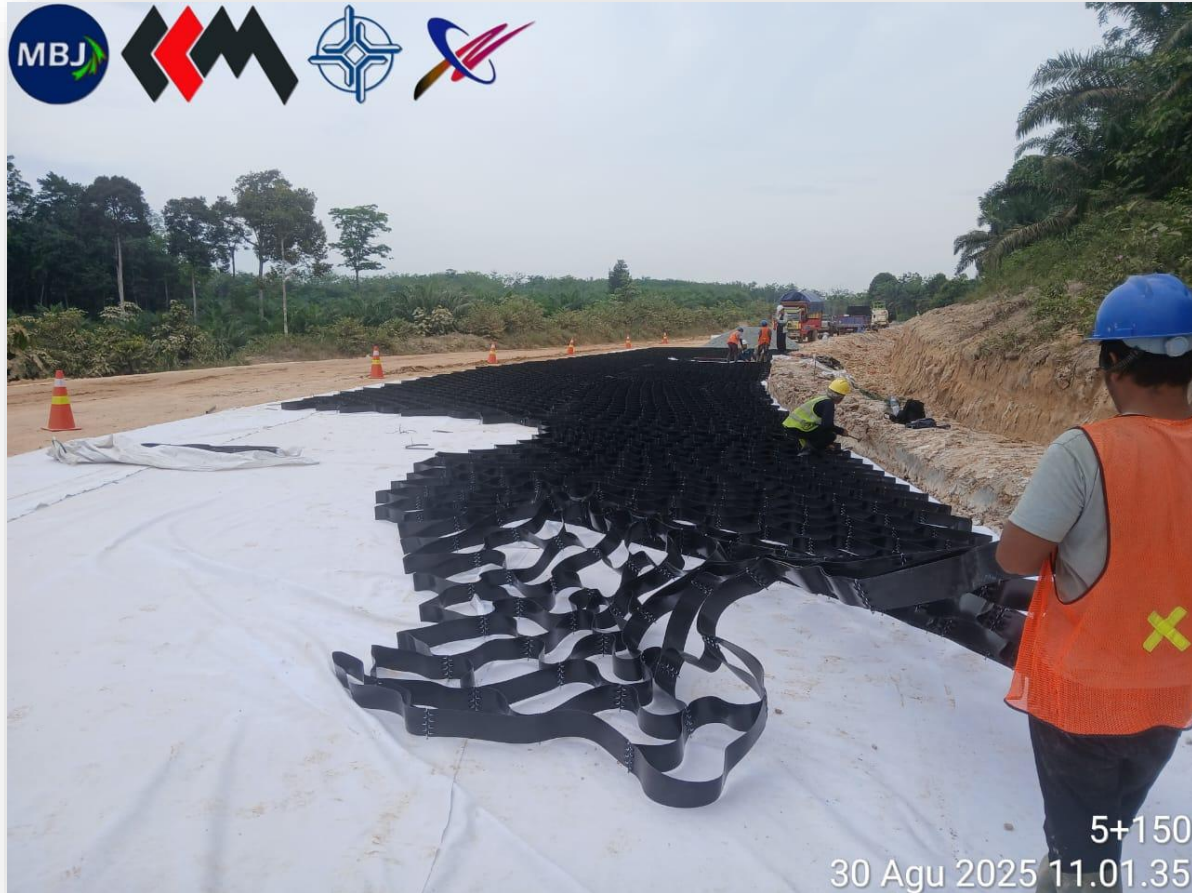
Road Construction Progress with Geo Grid
