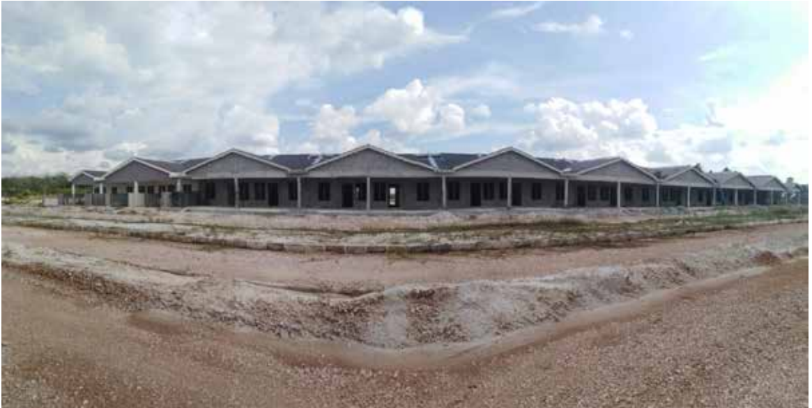
Sri Iskandar's terrace houses in progress
