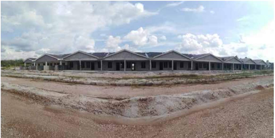
Sri Iskandar's terrace houses in progress
