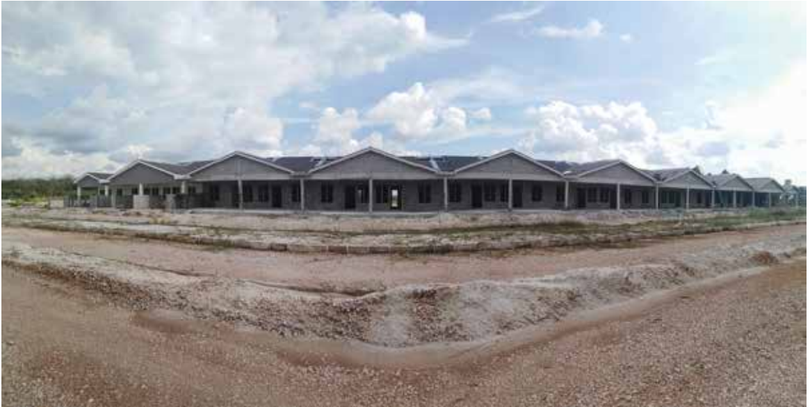
Sri Iskandar's terrace houses in progress
