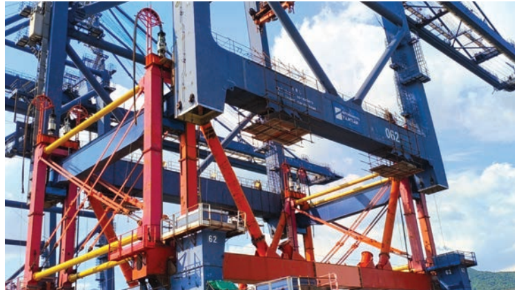
Quay crane heightening at YANTIAN.
