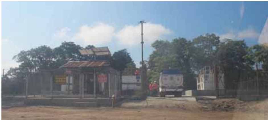
Figure 8-16 Fuel Storage Compound
