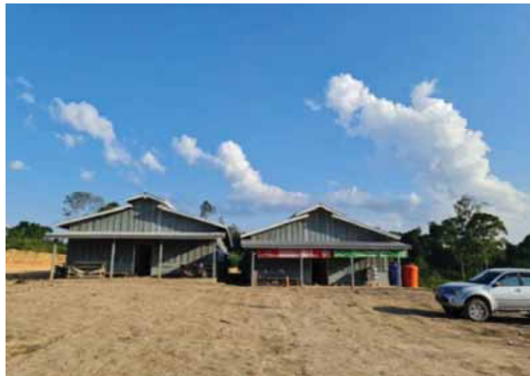
Figure 8-14 Contractor Messing and Office
