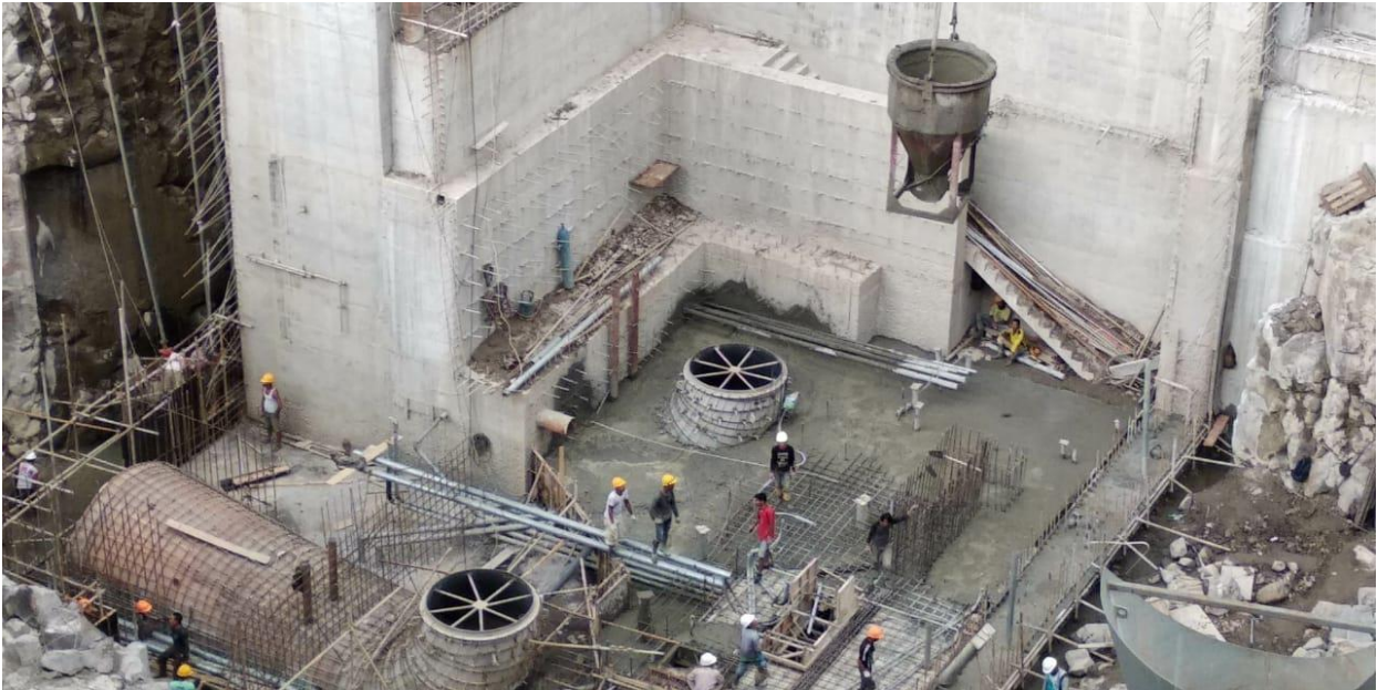
Workers putting together Aenergy’s mini-hydropower plants in North Sumatra.
