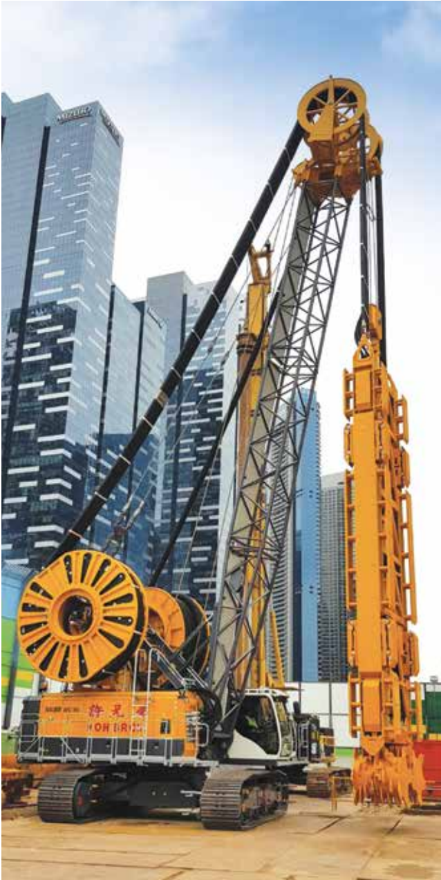
100m-Trench Cutter used at MRT Circle Line 6
