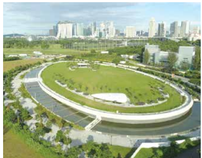
Marina East Desalination Plant
