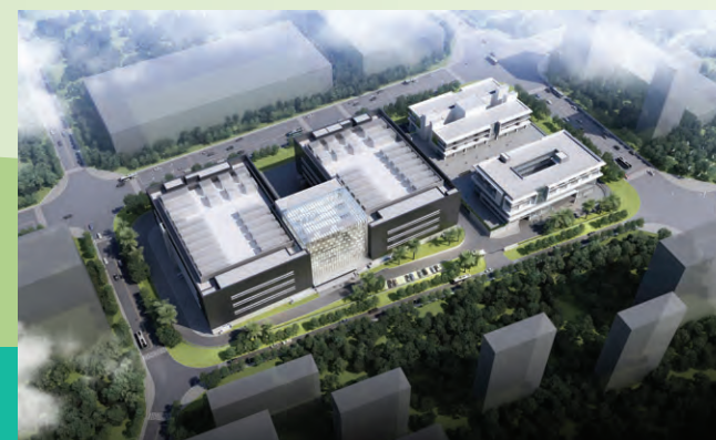
Data centre in Huizhou, China
