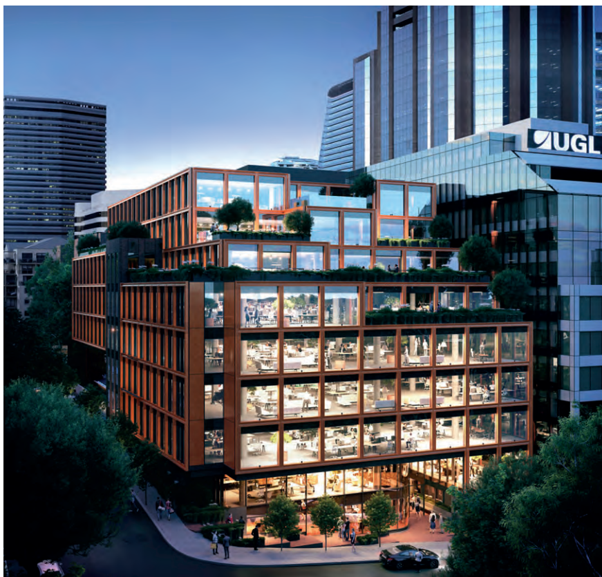
Keppel REIT's sustainable Grade A office building, Blue & William, which is under development in North Sydney, is designed to achieve the 5 Star Green Star Design and As Built Rating by the Green Building Council of Australia, as well as the 5.5 Stars National Australian Built Environment Rating System Base Building Energy Rating.
