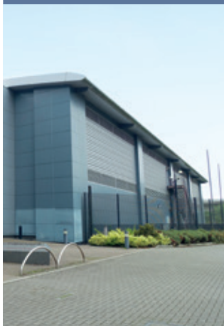
Cardiff Data Centre
