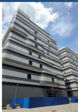
Guangdong Data Centre 3
