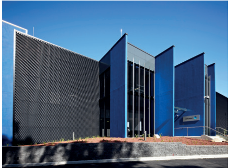
Intellicentre Campus is located within Macquarie Park in the north of Sydney, and is 12km away from the central business district.
