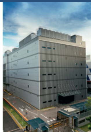
Keppel DC Singapore 3
