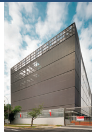
Keppel DC Singapore 4
