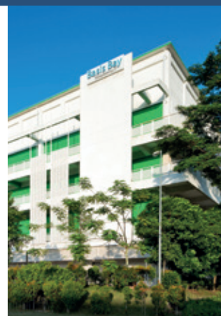
Basis Bay Data Centre
