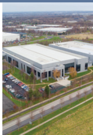
Keppel DC Dublin 1
