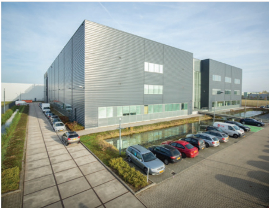
Keppel, together with its private funds, has more than $2 billion worth of data centre assets under development and management that Keppel DC REIT can potentially acquire.
