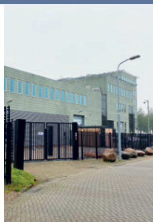
Amsterdam Data Centre
