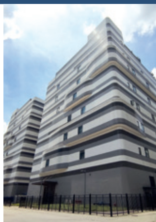
Guangdong Data Centre 2
