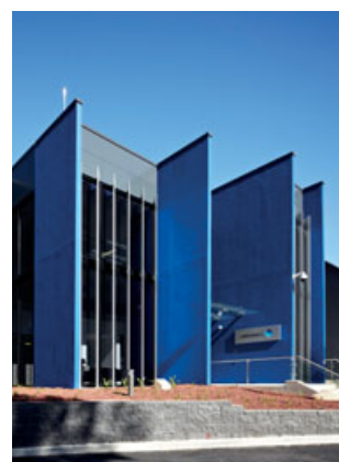
Intellicentre 2 Data Centre
