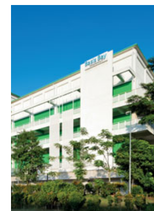
Basis Bay Data Centre
