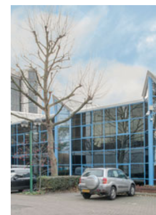
GV7 Data Centre
