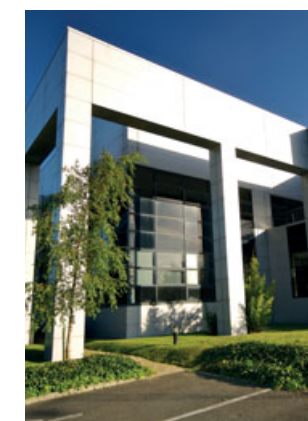
Keppel DC Dublin 1
