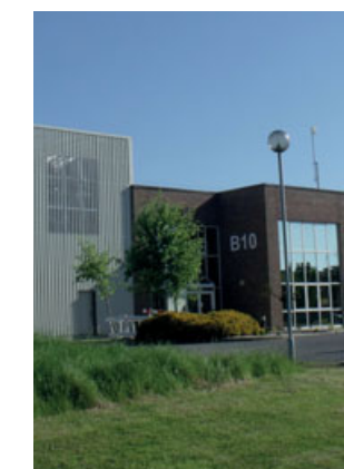
Keppel DC Dublin 2
