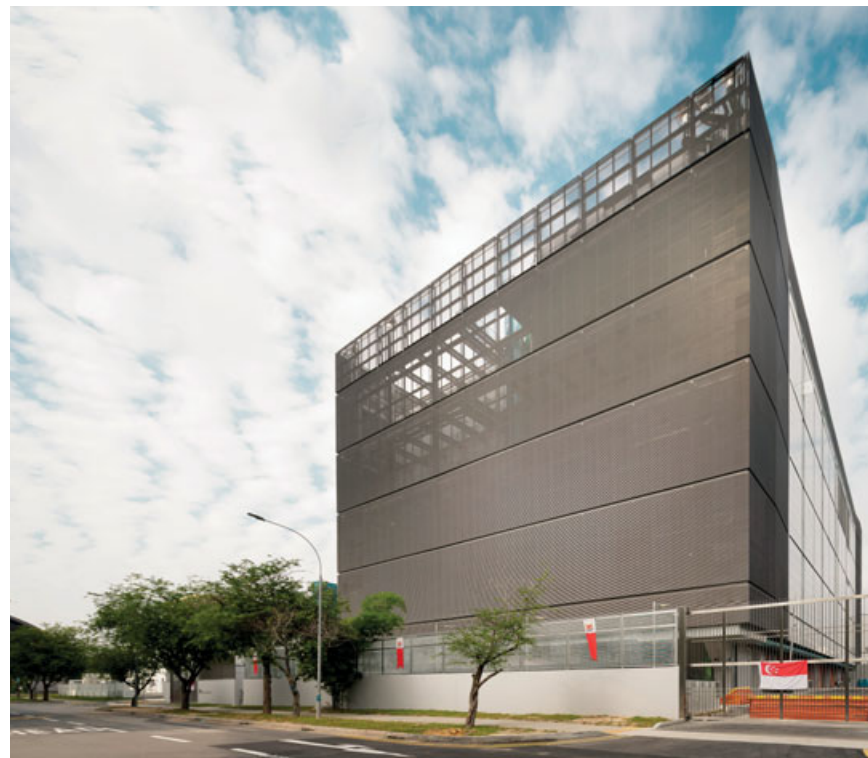
Strengthened Singapore footprint with strategic acquisitions of Keppel DC Singapore 4 (in image) and DC1.
