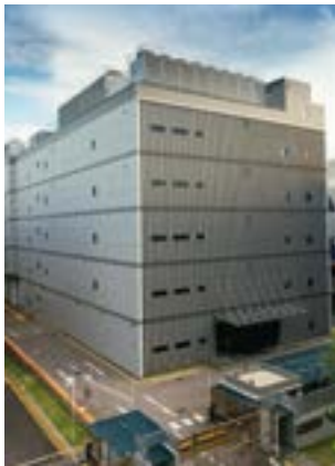
Keppel DC Singapore 3
