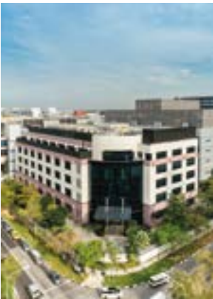
Keppel DC Singapore 1
