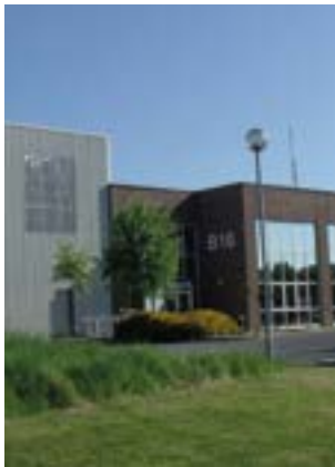
Keppel DC Dublin 2
