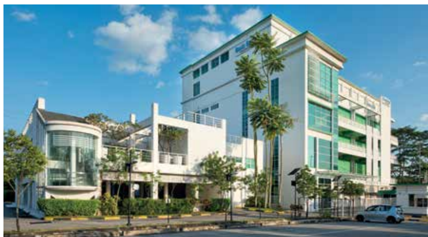
Basis Bay Data Centre in Cyberjaya, Malaysia.
