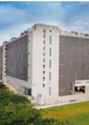
Keppel DC Singapore 5
