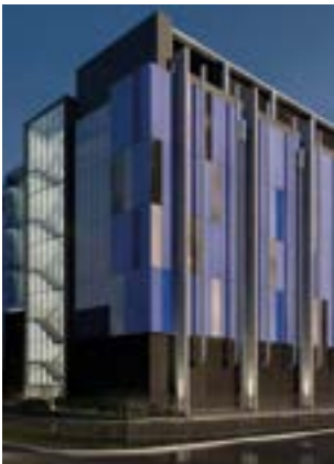
Intellicentre 3 East Data Centre (Under development)
