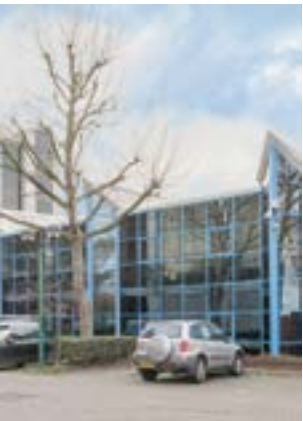
GV7 Data Centre
