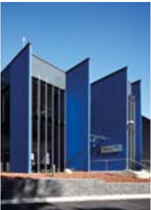
Intellicentre 2 Data Centre
