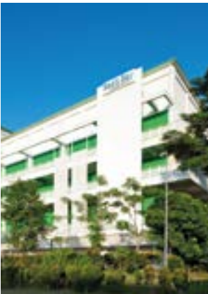
Basis Bay Data Centre
