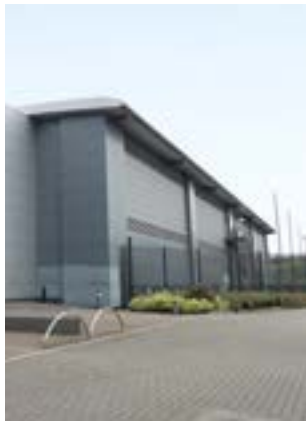
Cardiff Data Centre
