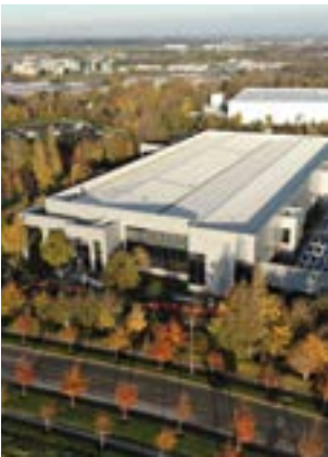
Keppel DC Dublin 1
