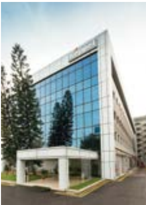
Keppel DC Singapore 2
