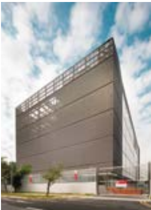
Keppel DC Singapore 4
