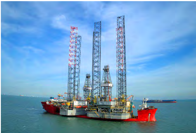
Rigs reactivation works
