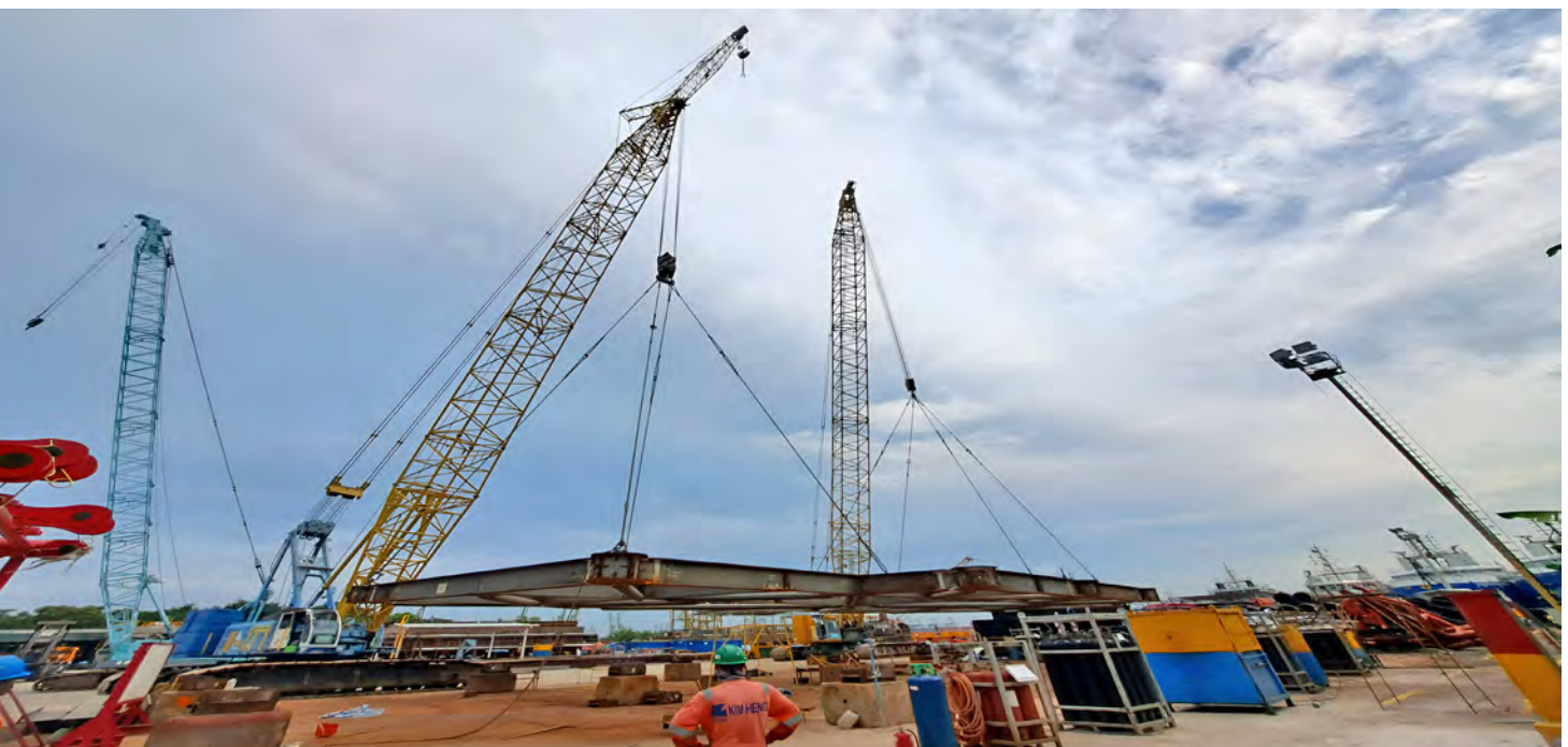
Steel modules ordered from Dyna-Mac under fabrications
