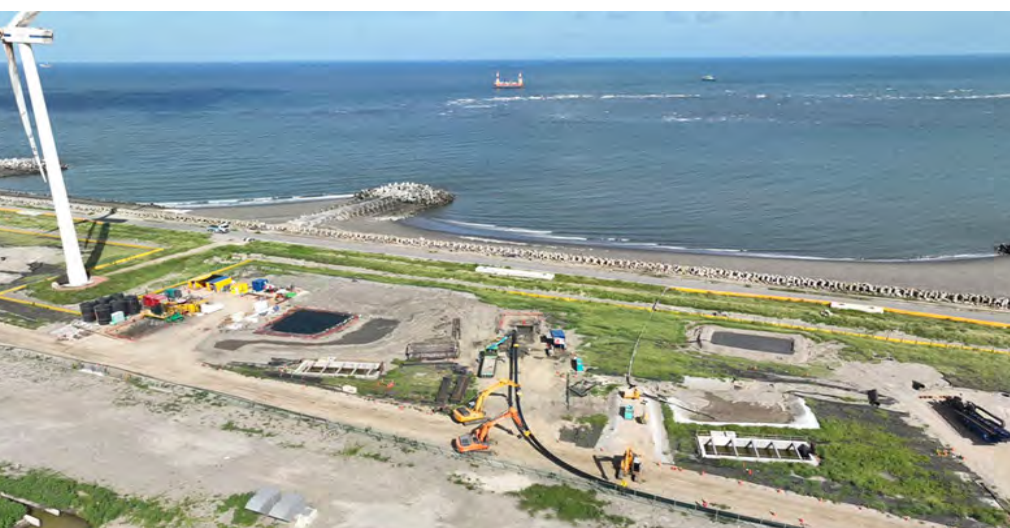
Hailong Offshore Wind Farm HDD works in Taiwan
