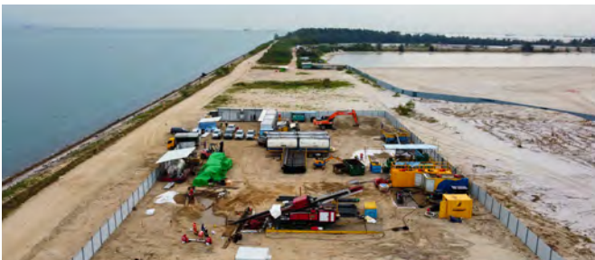
Bifrost submarine fibre optic cable HDD works in Tuas
