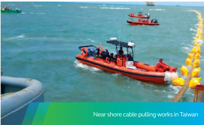
Pipe conduit pullback operation in Yulin, Taiwan
