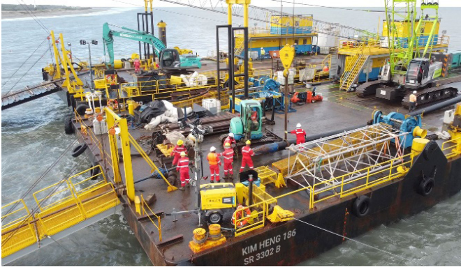
Pipe conduit pullback operation in Yulin, Taiwan
