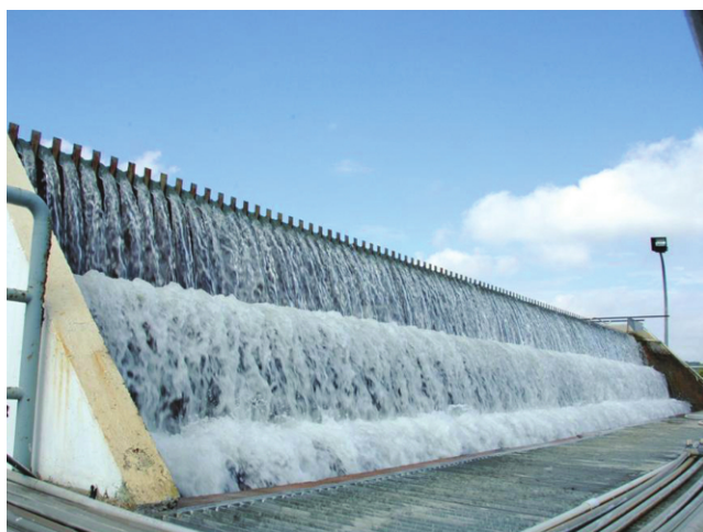
Figure 4. Aeration process at the Batam WTP
