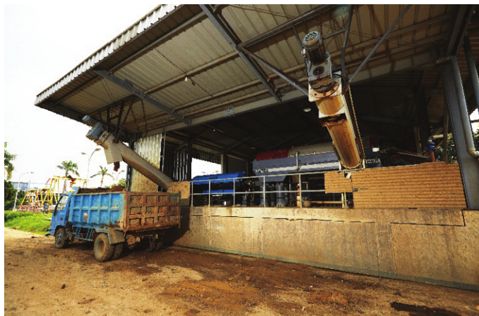
Figure 5. Sludge dewatering system
