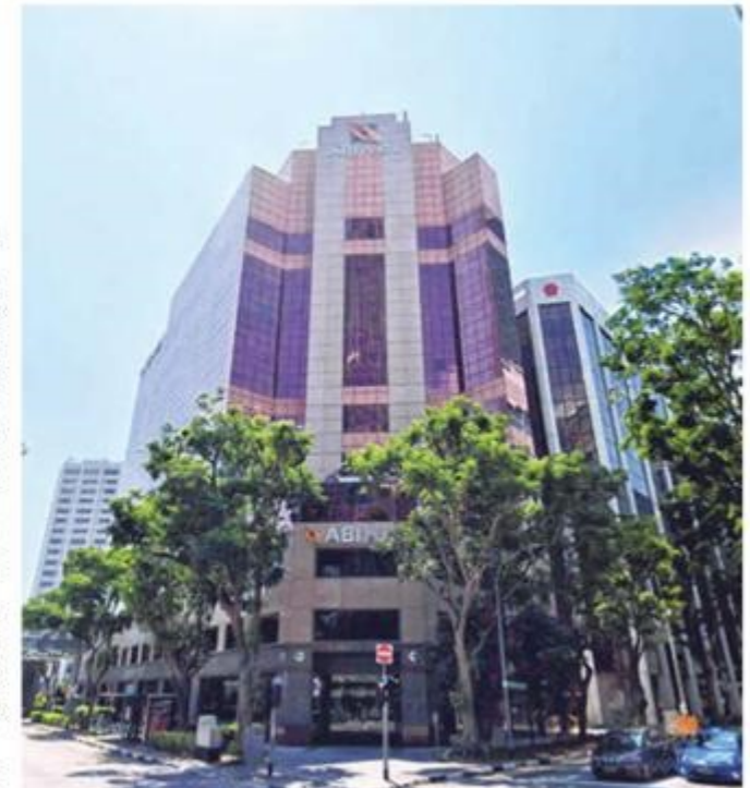
ABI Plaza, with triple frontages on Keppel, Tanjong Pagar and Lim Teck Kim roads, is owned by listed MYP, which paid S$175 million for the freehold property in 2011. PHOTO: GOOGLE MAPS
