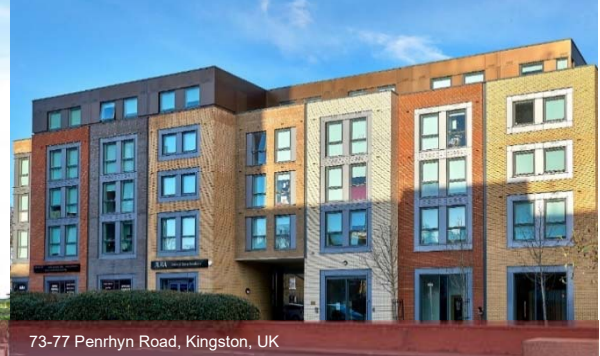
73-77 Penrhyn Road, Kingston, UK
