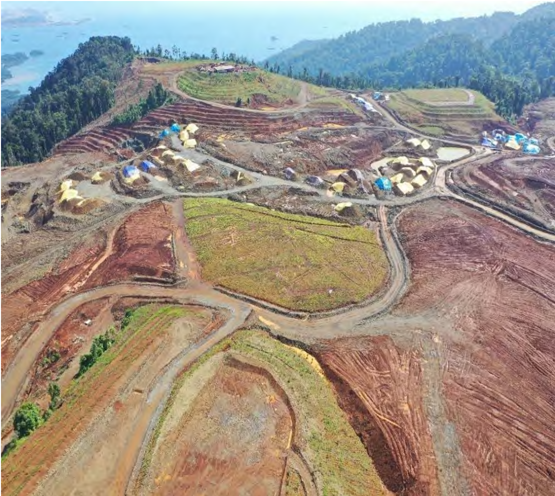
Photo 1 Mine rehabilitation progress at Bete Bete pit
