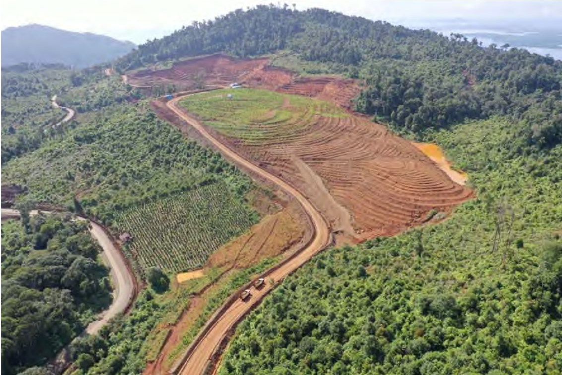
Photo 33 Central East pit 2022 (Source; Hengjaya)
