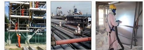
Scaffolding, Insulation, & Painting
