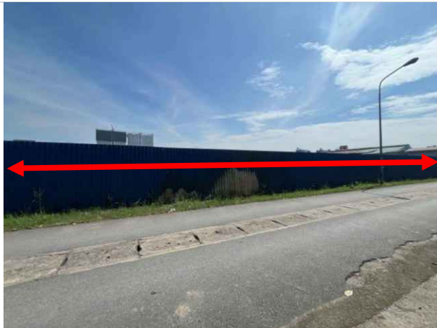
The Subject Property overview from Vinh Phu 13 Street
