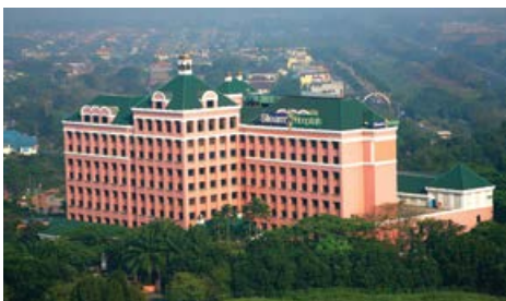
Siloam Hospital Lippo Village, part of First REIT's portfolio
