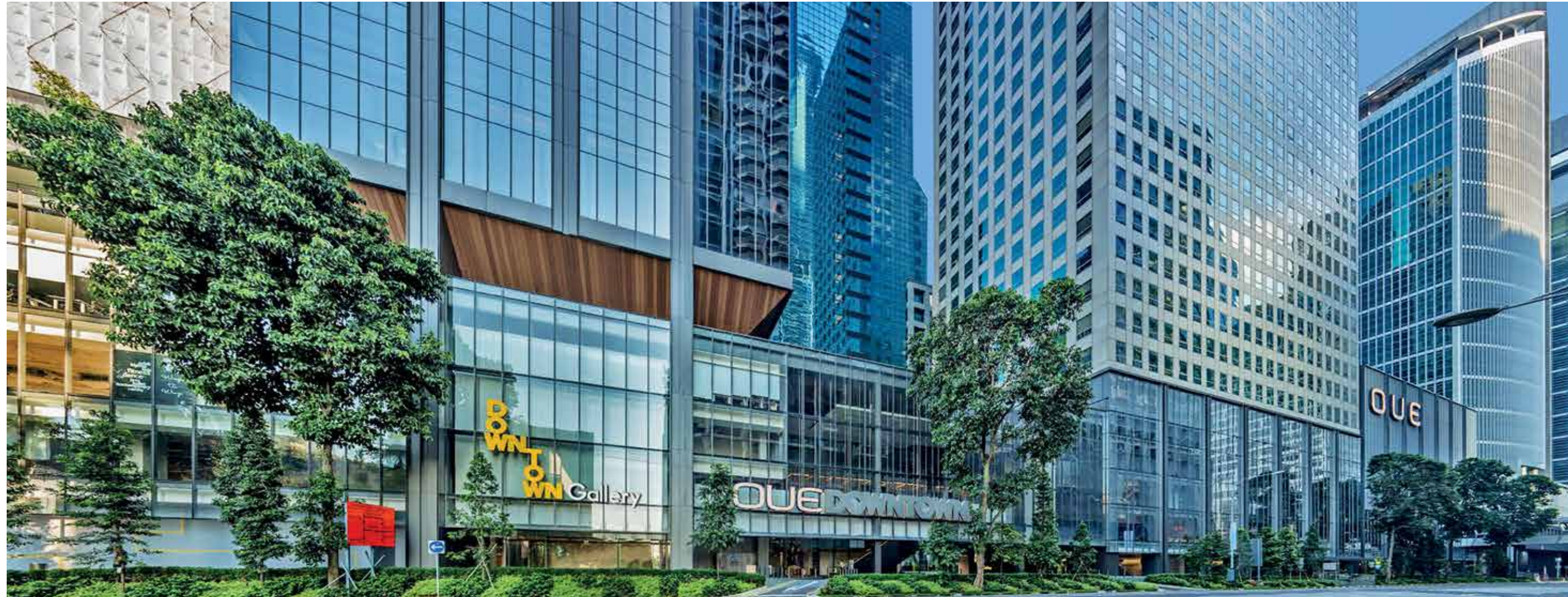
01 OUE Downtown is fronted by a 262-metre-wide pedestrian walkway along Shenton Way 02 Two towers of premium office space integrated with a vibrant retail mall
