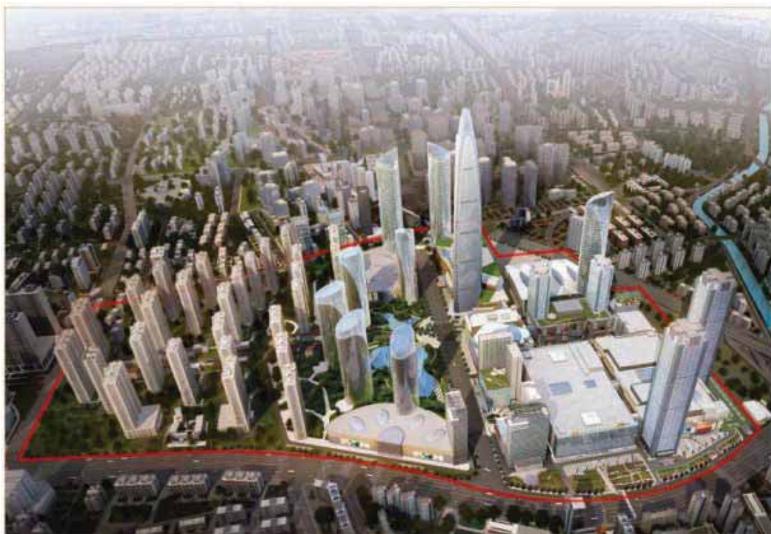
Figure 4.1 — Longemont Mixed Use Development
