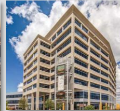
VILLAGE CENTER STATION I Denver, Colorado
