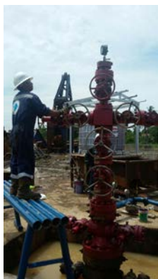
CLS-I TW wellhead opened
