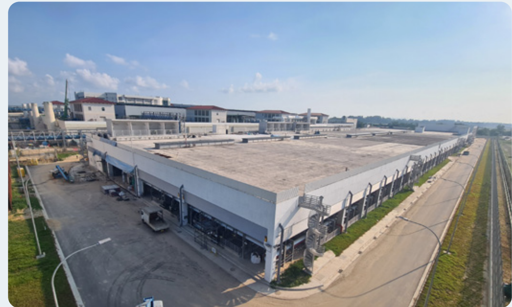
Rooftop of Changi Water Reclamation Plant where CNF3 will be situated.
