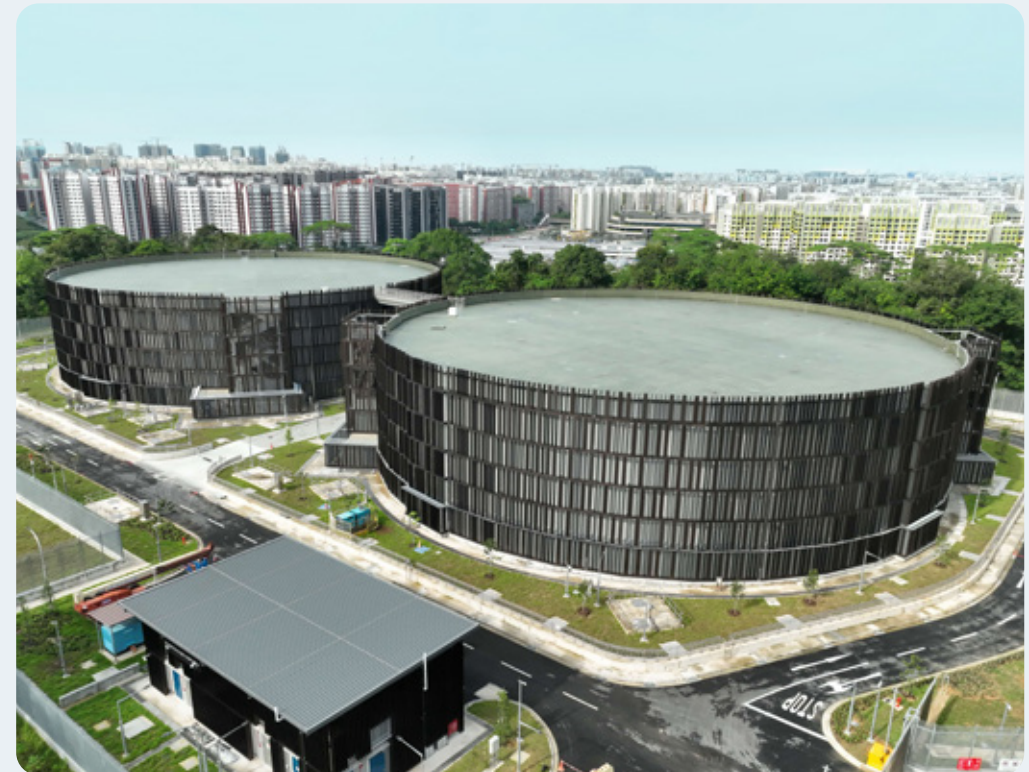
Aerial shot of Tengah Service Reservoir at Bukit Batok Road.
