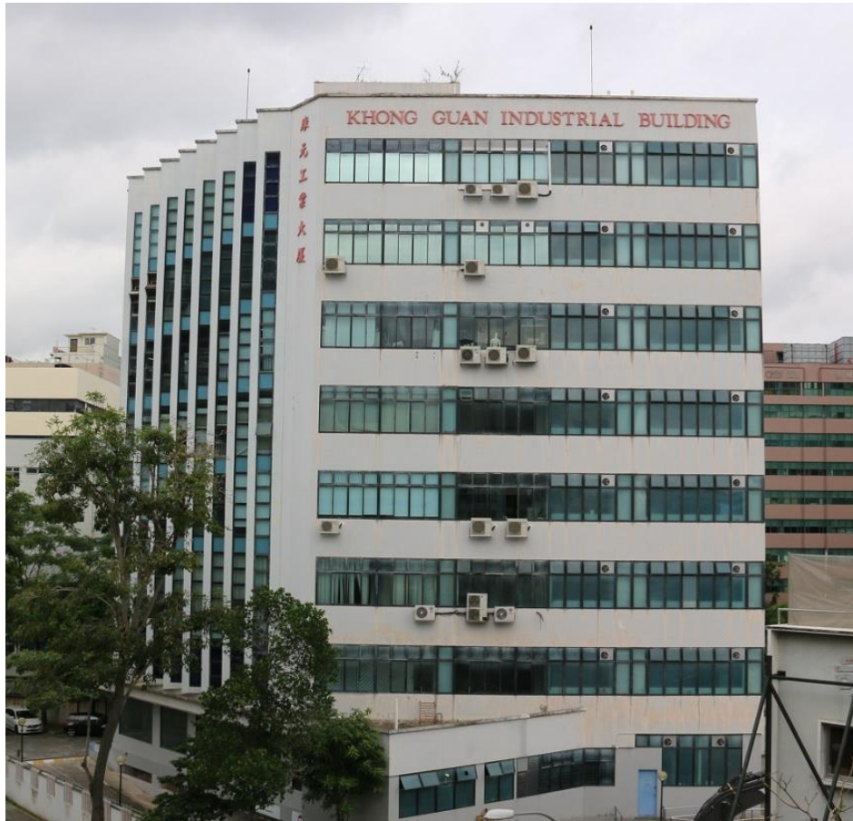
Figure 1 – Khong Guan Industrial Building at 20 Mactaggart Rd
