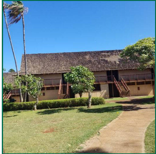
Shuttered Kaluakoi Hotel Structures
