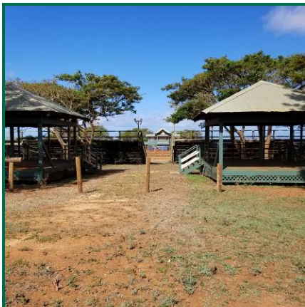
Rodeo Facility near Maunaloa
