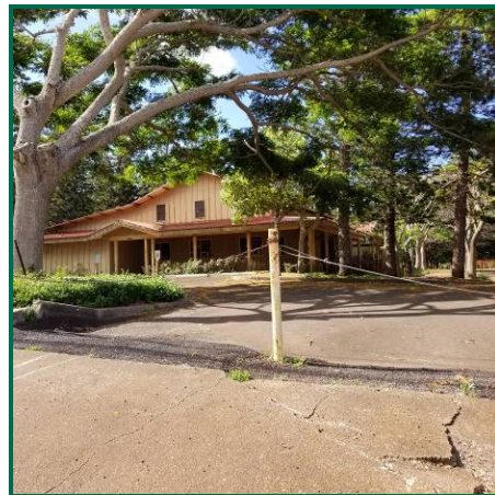
Existing Warehouse near Lodge
