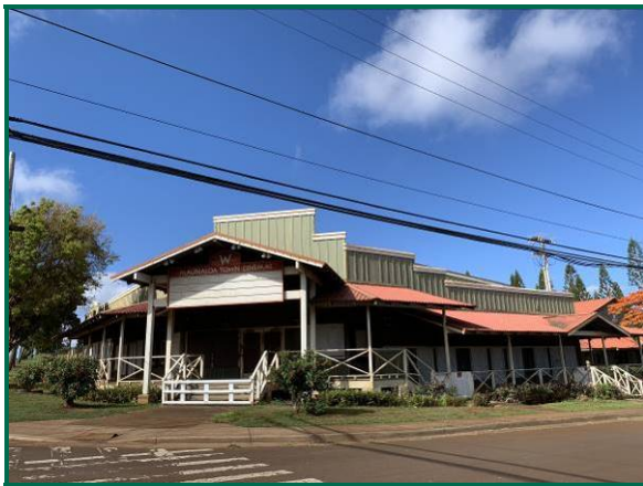
Shuttered Theater Building
