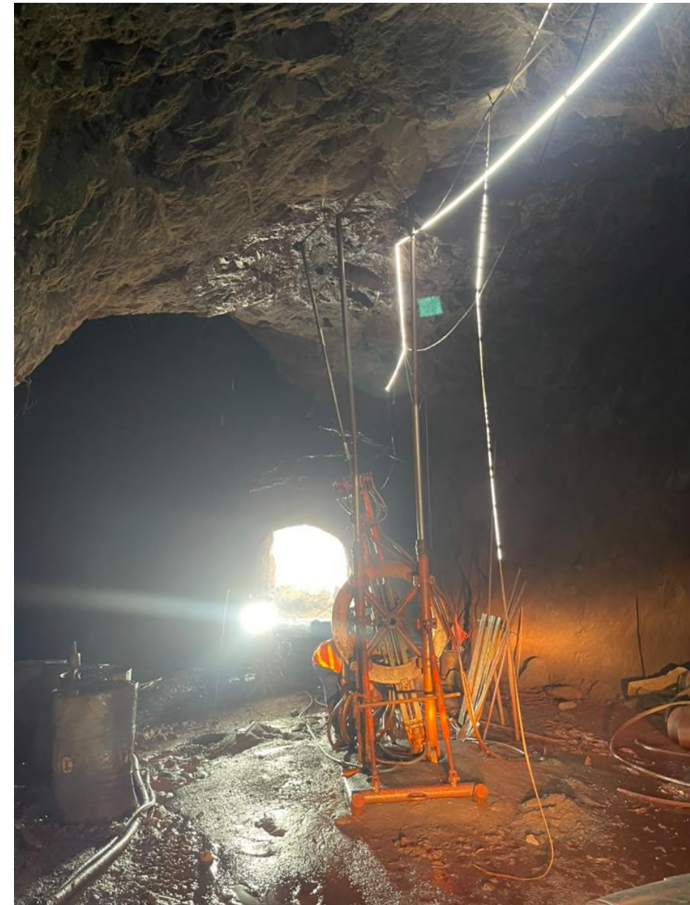
Underground Stopping Drilling
