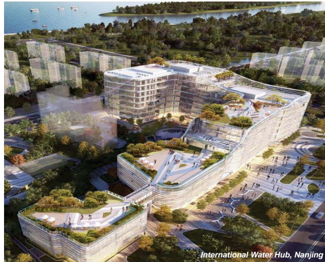
International Water Hub, Nanjing
