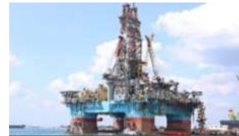
Offshore rig repairs
