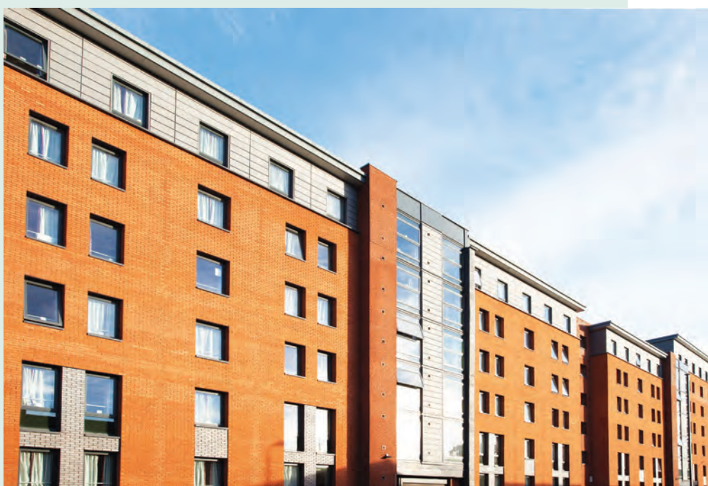
PBSA: external facade of Central Quay, Sheffield
