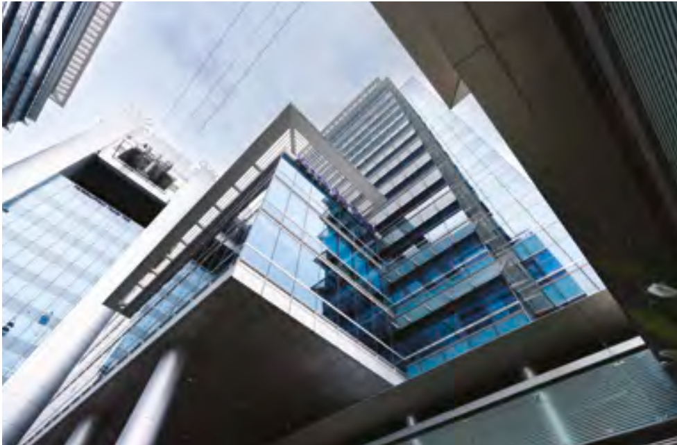
Keppel Bay Tower is the first commercial building in Singapore to be certified by the BCA as a Green Mark Platinum (Zero Energy) building. PV panels installed on the roof of the building can generate an energy yield of about 100,000 kWh per annum.
