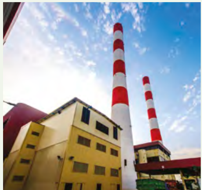
Senoko WTE Plant
