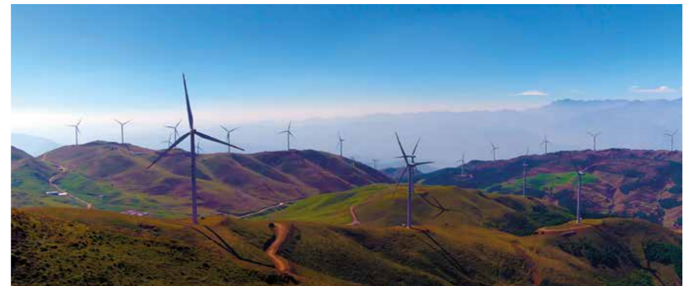
Sembcorp wind assets in Yunnan, China
