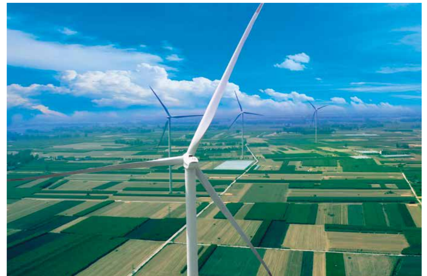
Sembcorp wind assets in Henan, China
