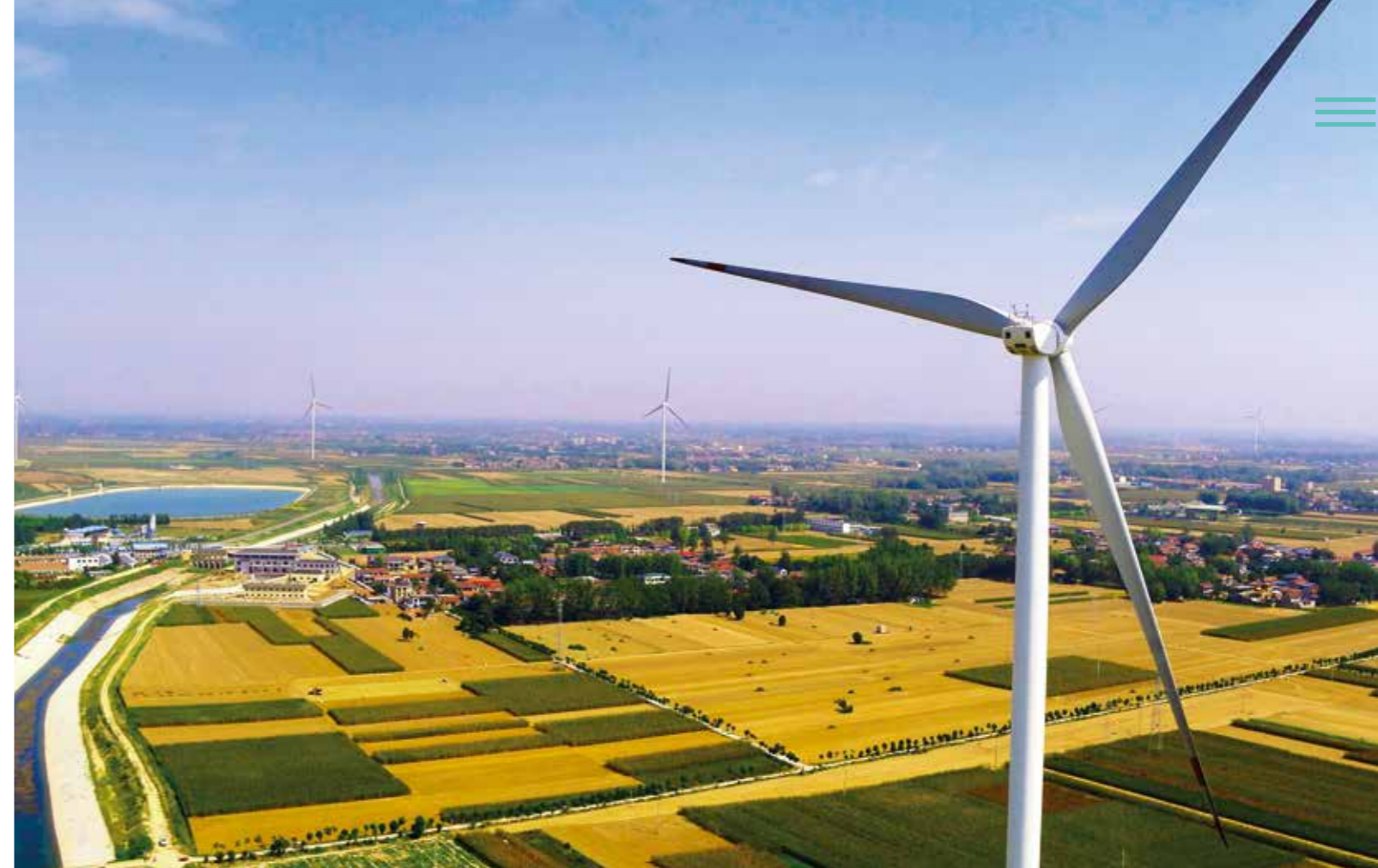
Sembcorp's wind asset located in Henan Province, China
