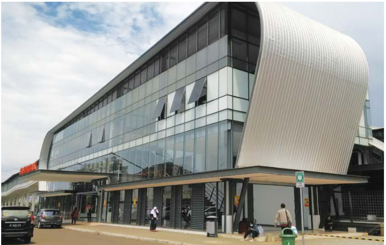
Revitalisation of the Cisauk Train Station
