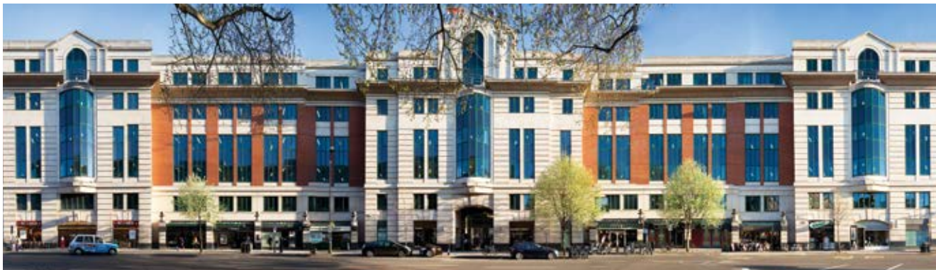
UK - 33 Horseferry Building
