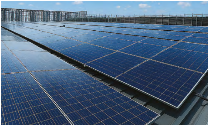
A rooftop solar photovoltaic system helps to support low-carbon operations at DC Tuas.
