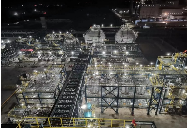
Night view of the completed Pp plant
