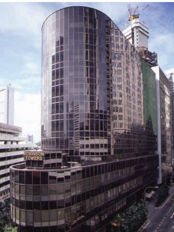
1980 Acquired Robinson Towers, Singapore
