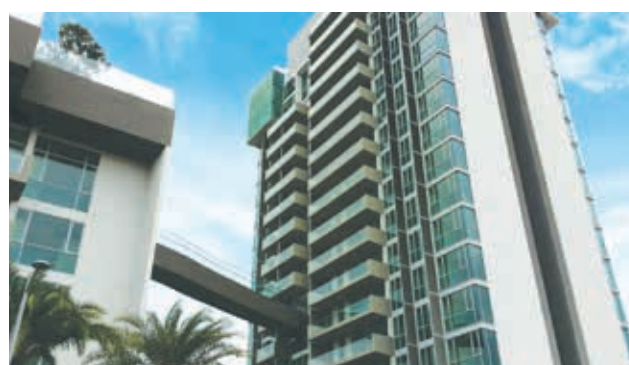
Sennett Residence, Singapore
