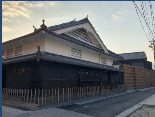
Ongoing Hotel AM project: Azumi Setoda
