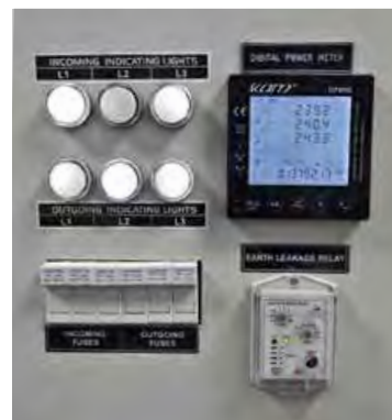
Electrical meters were installed at every level in SETSCO's building to monitor electricity consumption.
