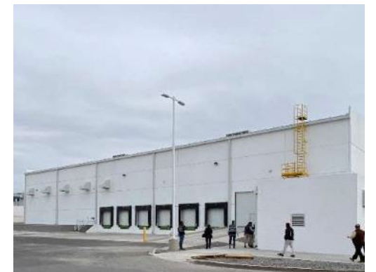
Warehouse, Dock & Label Printing Room
