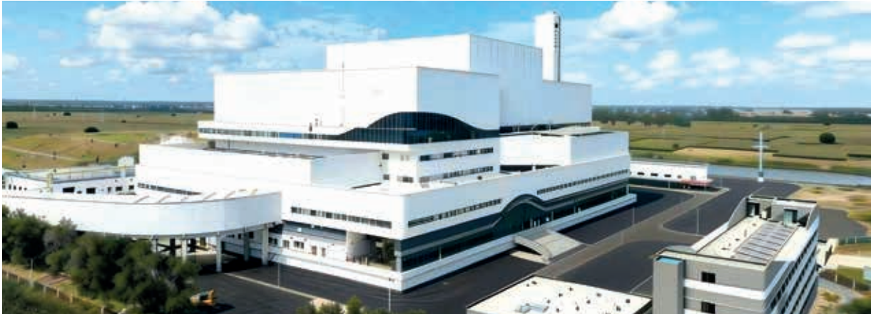
Figure 4: Panoramic view of Baoding Jinhuan WTE Facility in Hebei Province 图 4：河北省高碑店垃圾发电项目全景图
