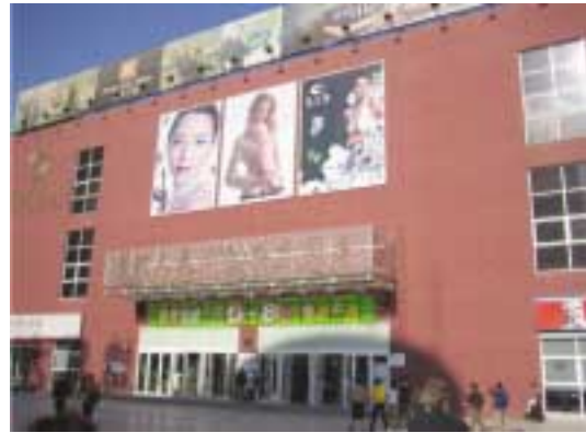
Photo 6.16 External view of Wu Mart Plaza
