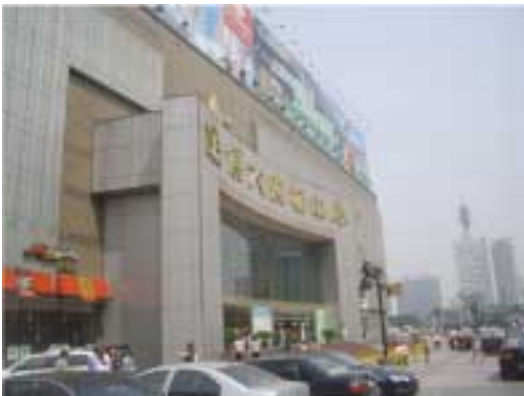
Photo 8.1 External view of entrance
