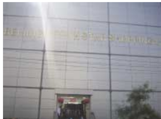
Photo 6.12 North Star Shopping Centre
