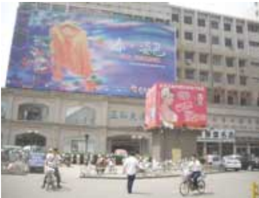
8.9 External view of Zhengzhou Department Store
