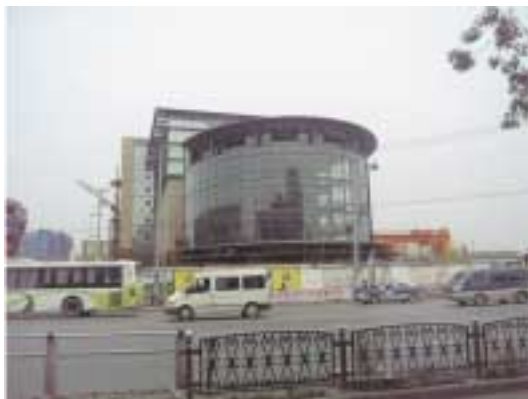
Photo 7.5 External view of Hui Heng Centre (expected completion 2007)
