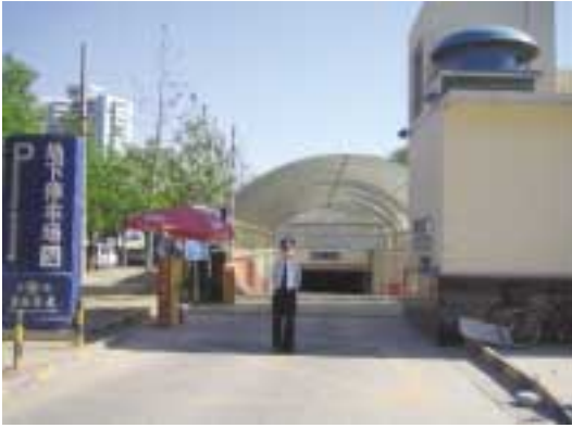
Photo 6.3 Entrance to underground carpark
