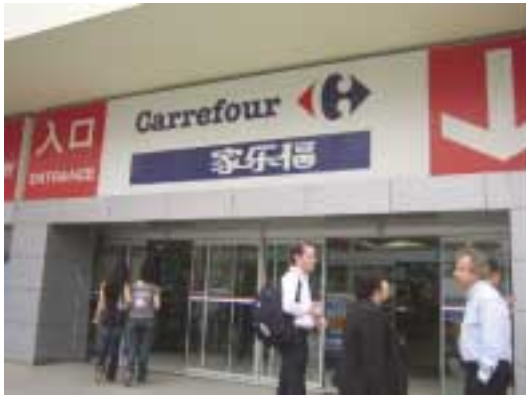
Photo 5.1 Main entrance to Jiulong Mall
