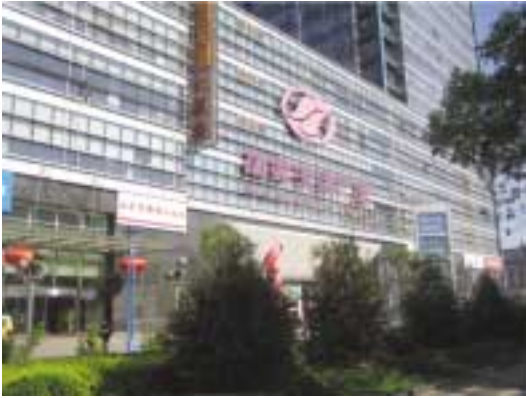
Photo 6.13 External view of Wu Mart Plaza
